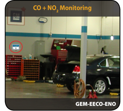
Repair Shops - Gas & Diesel Engine Exhaust
